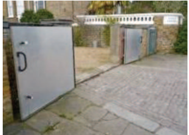
Above: Example of a flood gate installed to a communal car parking area
