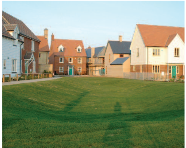
Infiltration basin in dry state, Ipswich
