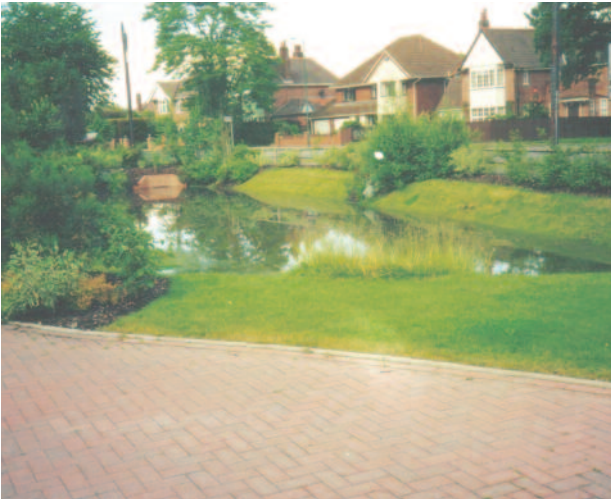
Detention Basin, Ipswich
